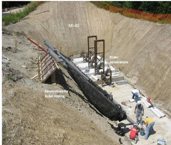
Figure 2: Installation of new kicker penetrations. The shielding has been removed to expose the Main Injector tunnel ceiling. Note gray penetration pipes.
