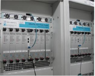
Figure 4: SPS/CPS power converter modules.
