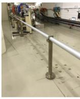
Figure 3: The support of isolation tube are adjusted and positioned on the exact location of ground in the straight section of TPS storage ring.
