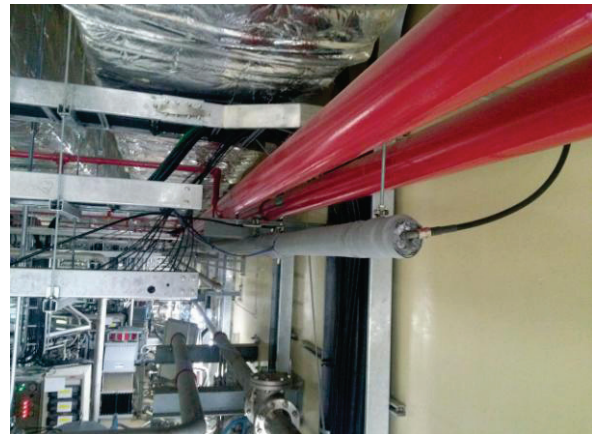
Figure 6: Temperature-controlled RF reference line.
