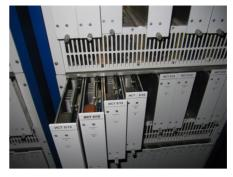
Figure 5: Programmed power supply sources of storage ring magnetic elements power supply control system.
