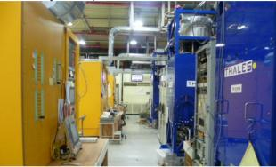
Figure 2: Three 300kW klystrons and KSUs.
