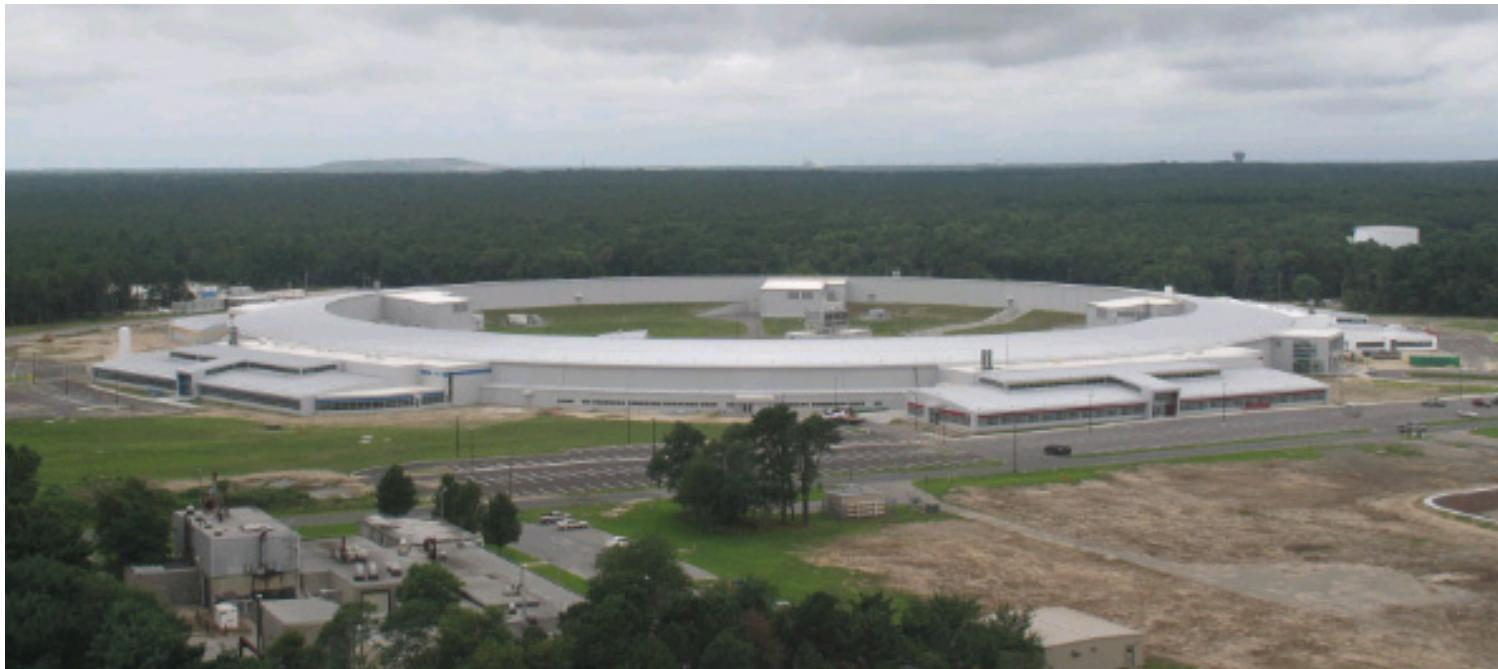
**General parameters:** 3 GeV, 500 mA; circumference: 791.5 m; lattice: 30 cell, DBA
