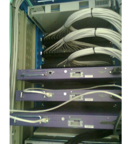
At the time of writing more than 110 peripheral switches, Summit X350 and X150 made by Extreme Networks, are installed in the 65 racks that host the control system and diagnostics devices, distributed along the FERMI buildings. A grand total of about 1800 devices are connected to the control system network.
