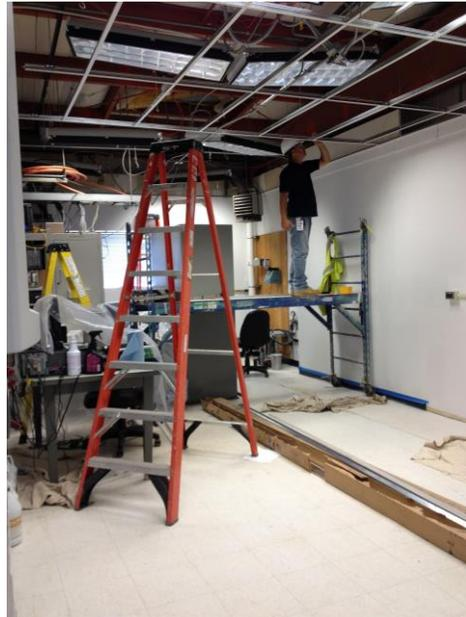
Figure 8: Photo of work in progress in the BLIP control room on September 8, 2014 where 7 new equipment racks will be installed to house the new electronics. Facilities work includes upgraded power, new ceiling and lighting, new air conditioning system, and cable trays.
