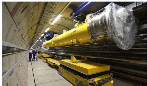
Figure 9: First E-XFEL accelerator module installed in the tunnel.
