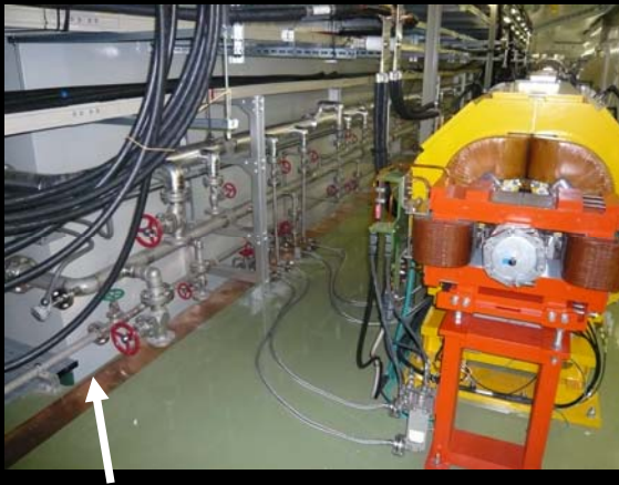
Grounding copper plate
