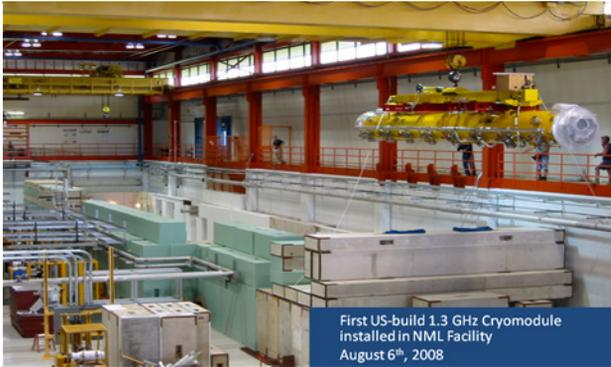
Figure 12: Installation of a US-assembled 8 cavity TESLA cryomodule in the New Muon Laboratory facility at Fermilab.
