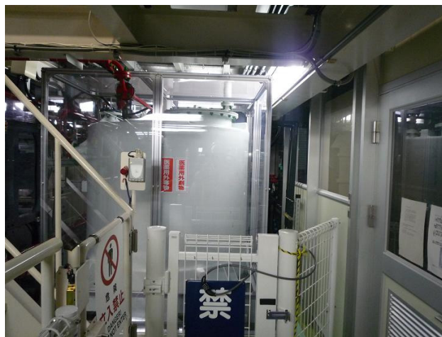
Figure 1: Reservoir tank of EP-electrolyte (2,000 L) in STF-EP facility at KEK.
