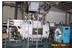
Fig.2 East cavity in BEPCII tunnel
