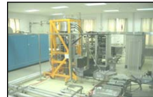
Fig.3 250KW (CW) klystron in East RF hall
