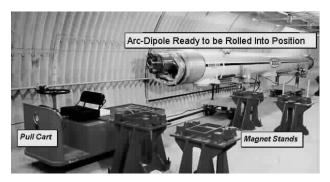
**Figure 3: Dipole Installation**
