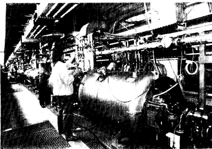
Fig. 2 - The first 4 cryostats installed in the HERA tunnel.
