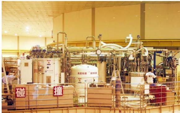
Figure 2: Cryogenic plant designed for srf module.
