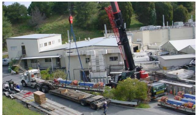
Figure 1: Removal of SPEAR 2 magnet/chamber girders.
