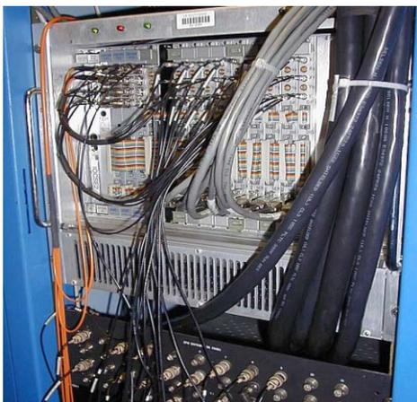
Figure 3: Filter and fan trays obstructed by cables.
