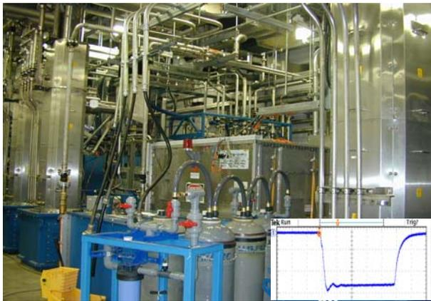
Figure 6: HVCML driving the RFQ and DTL 1 klystron (402.5 MHz, 2.5 MW) installed in the klystron gallery. The graph shows the flat top of a full 1.3-ms-long pulse.
