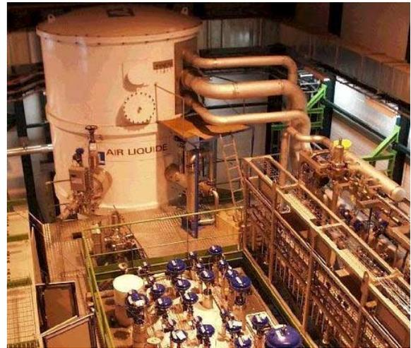
Figure 2: Coldbox of the new 18 kW refrigerator (4.5 K).
