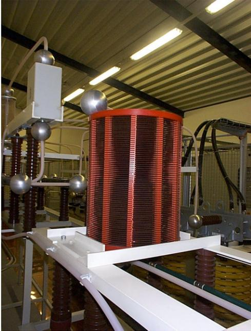
Fig 2. High voltage inductor on output of Jaeger HVPC
