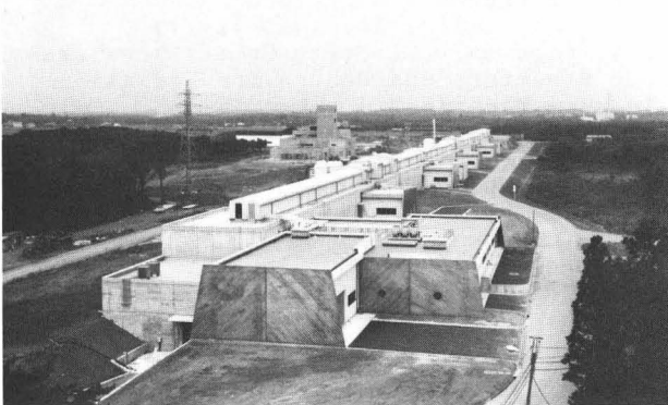
Fig. 1 Building of the PF Linac.
