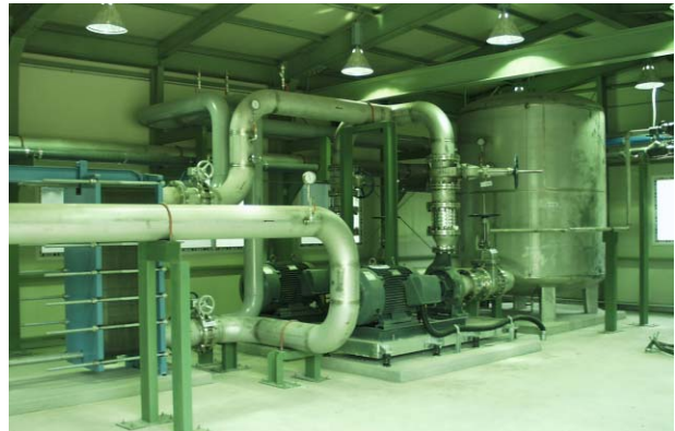
Figure 5: 2 MW DI water cooling system
