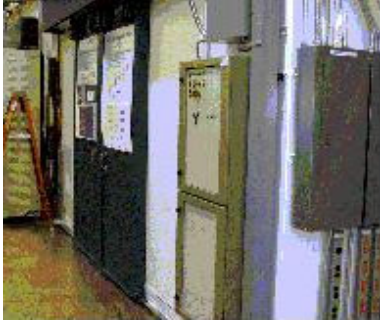
Fig. 1 Personnel Safety System (PSS)
