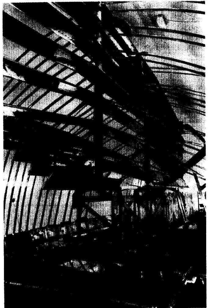
Construction of the Vivitron. The discrete electrodes.
