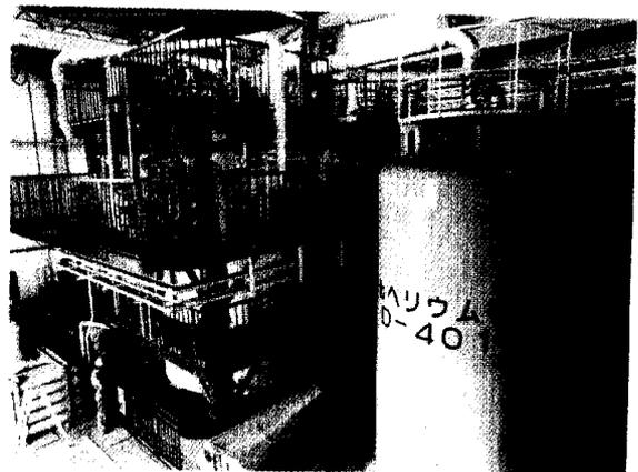
Fig. 8 Cold box (6.5 kW) for the TRISTAN superconducting RF cavity system.
