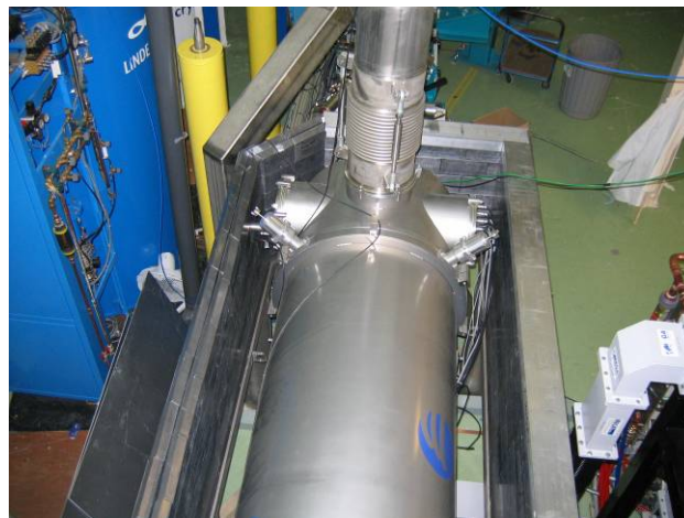
Figure 2: Lead shielding around the linac module under construction.
