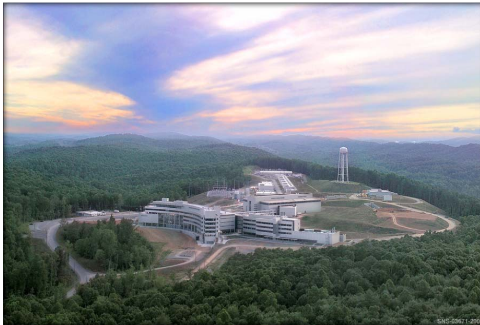
Figure 1: Overview of the construction site with accelerator systems, target buildings, the central laboratory office, JINS, CNMS and several support buildings overlaid on a early site photo on top of Chestnut Ridge at Oak Ridge National Laboratory.
