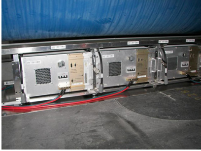
Figure 3: LHC60A frame under dipole cryostat.
