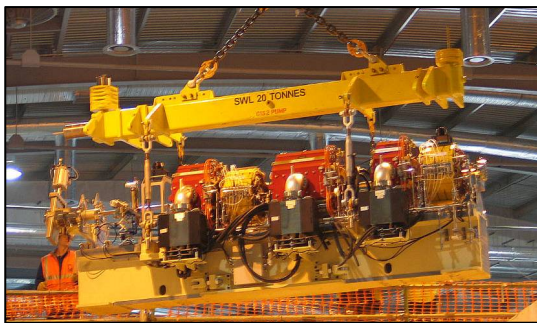
Figure 1 one Diamond girder assembly in the way to the tunnel.
