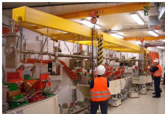
Figure 3 installation of complete sector inside the tunnel of the Australian Synchrotron
