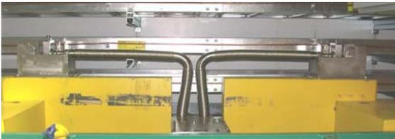
Figure 3: Double Contained Co-Axial Piping System
