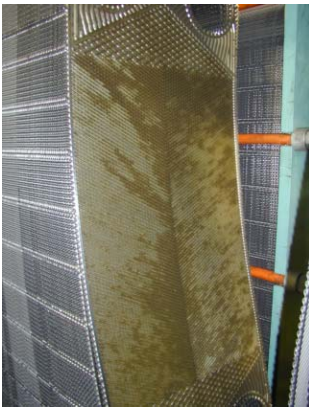
Figure 3: Dirty heat exchanger plate
