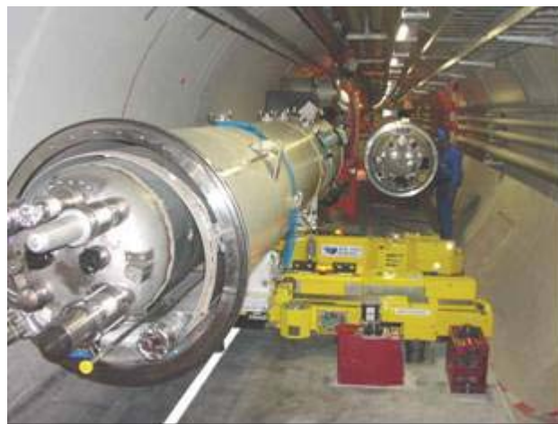
Figure 3: Transfer with TES of a short straight section to the magnet support jacks. In the background a cryo-dipole already in its tunnel position
