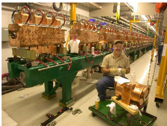
Figure 7: CCL bridge coupler installation preparation.
