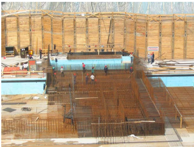
Figure 3: Preparation work for the gantry floor (06/04)
