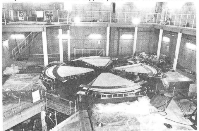
Fig. 2. A photograph of the sector magnets which are under installation in the cyclotron vault.
