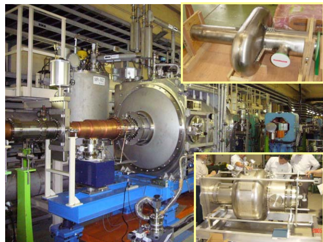
Figure 3: Installed crab cavity.
