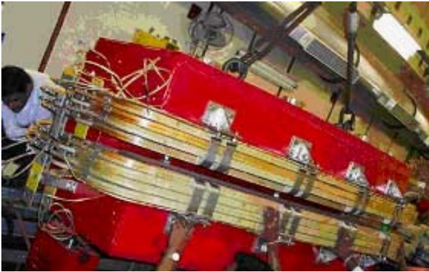
Figure 1: Installation of ring dipole at location.
