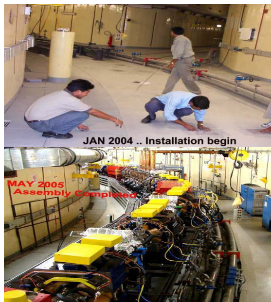
Figure 3: Beginning and completion of assembly.
