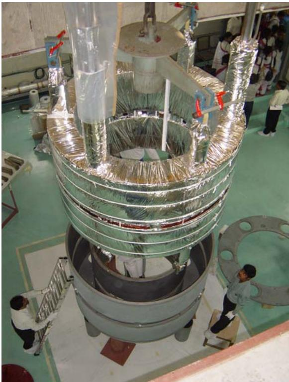
Figure 7: The insulated cryostat bobbin and LN2 shield assembly is being installed within the iron vacuum chamber (Coil Tank).
