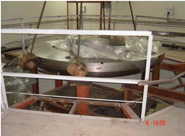
Figure 2: Main magnet pole base mounted on the pier support in the cyclotron building.
