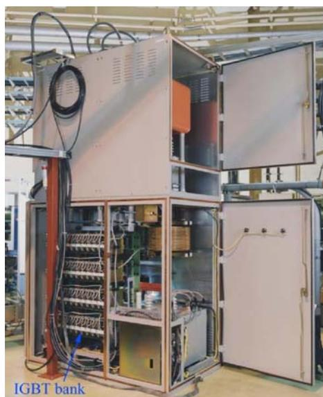
Figure 2: High voltage cabinet of the new klystron power supply
