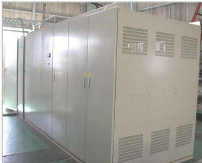
Figure 2: Power supplies for rf amplifier.
