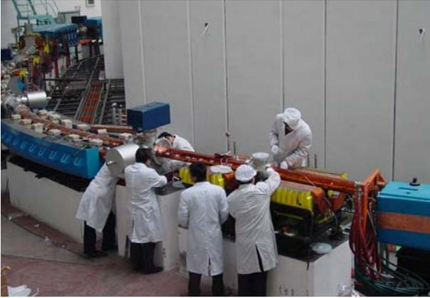
Figure 5: CSRm vacuum system is being installed
