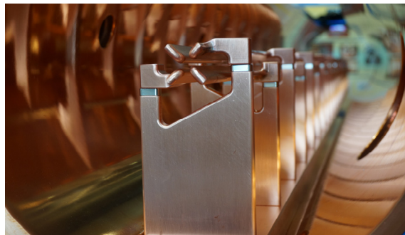
Figure 6: The 4 – Rod – RFQ during installation work.
