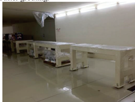
Figure 7: The injection girders were installed in the tunnel of TPS.
