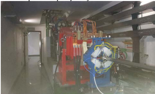
Figure 2: Injection bump of HLS II injector.
