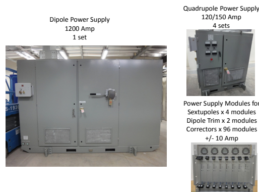
Figure 1: Large and medium/small power supplies for the dipole, quadrupole and correctors of TPS booster synchrotron respectively.
