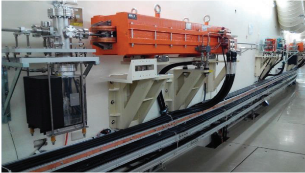
Figure 7: TPS BR installation status.
