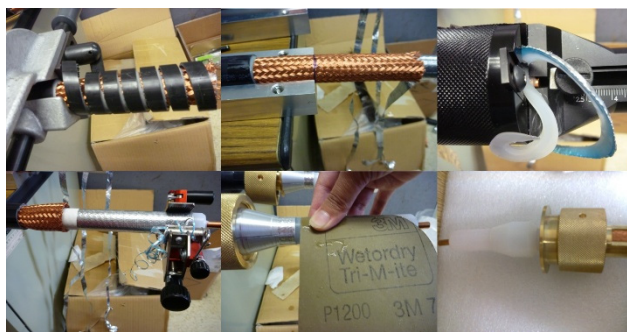
Figure 10: Steps to prepare a cable termination: upper, steps 1 to 3 (right); lower, steps 4 to 6 (right).
