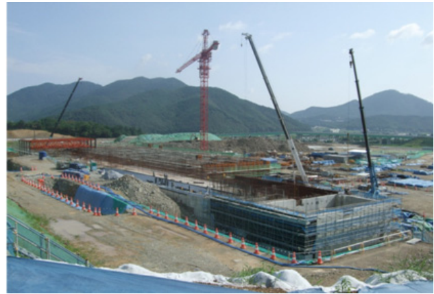
Figure 7: Construction of the accelerator building (July 31, 2011).
