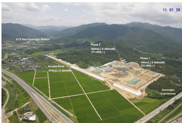
Figure 6: Bird's eye view of the construction site (July 29, 2011).
